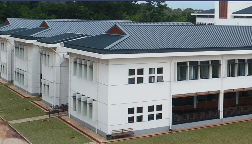
Shading facade of the outpatient building
