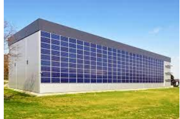
Building Integrated PV
