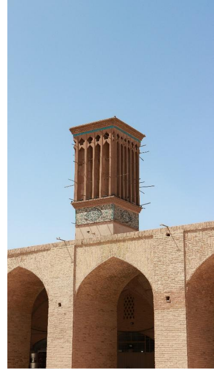
Traditional wind tower
