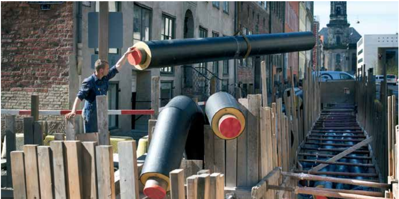
Figure 10: Installing new DH pipes in Copenhagen
