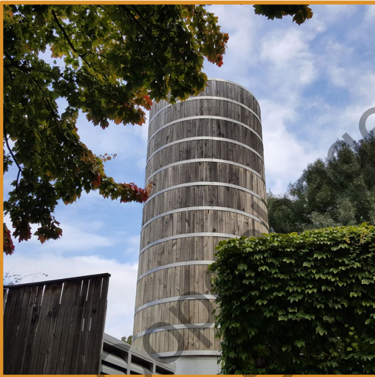
Source: Bunhill CHP plant in Islington, London. The tower is a large heat storage unit that reduces the need to provide heat from the district heating system', lanvisits
