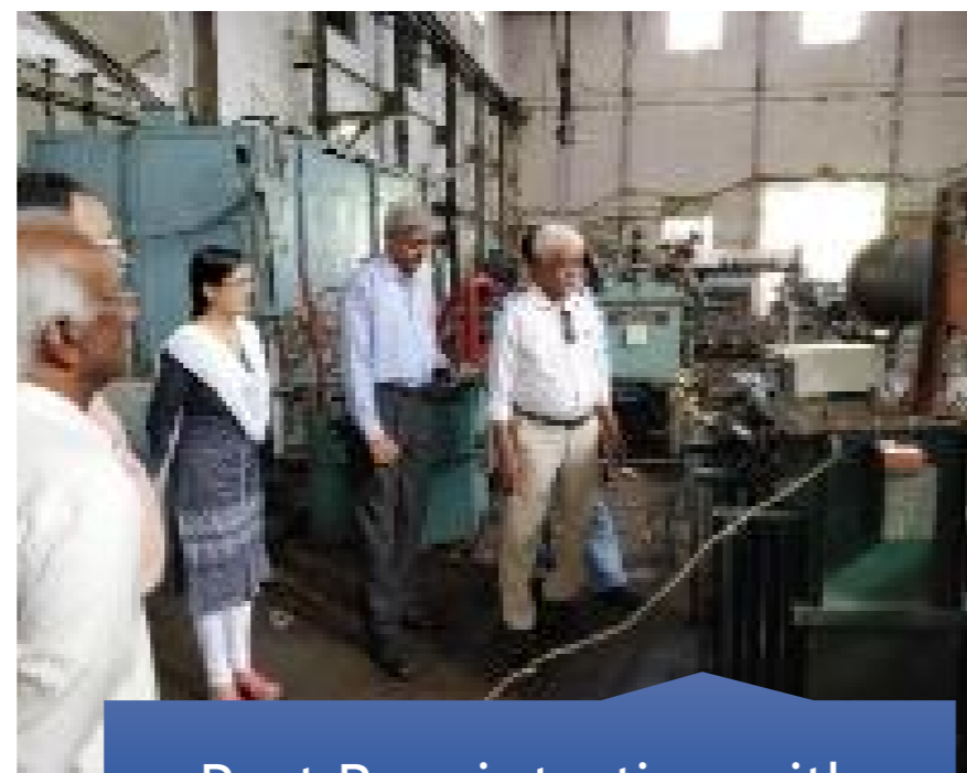
Post Repair testing with MPPKVCL representatives
