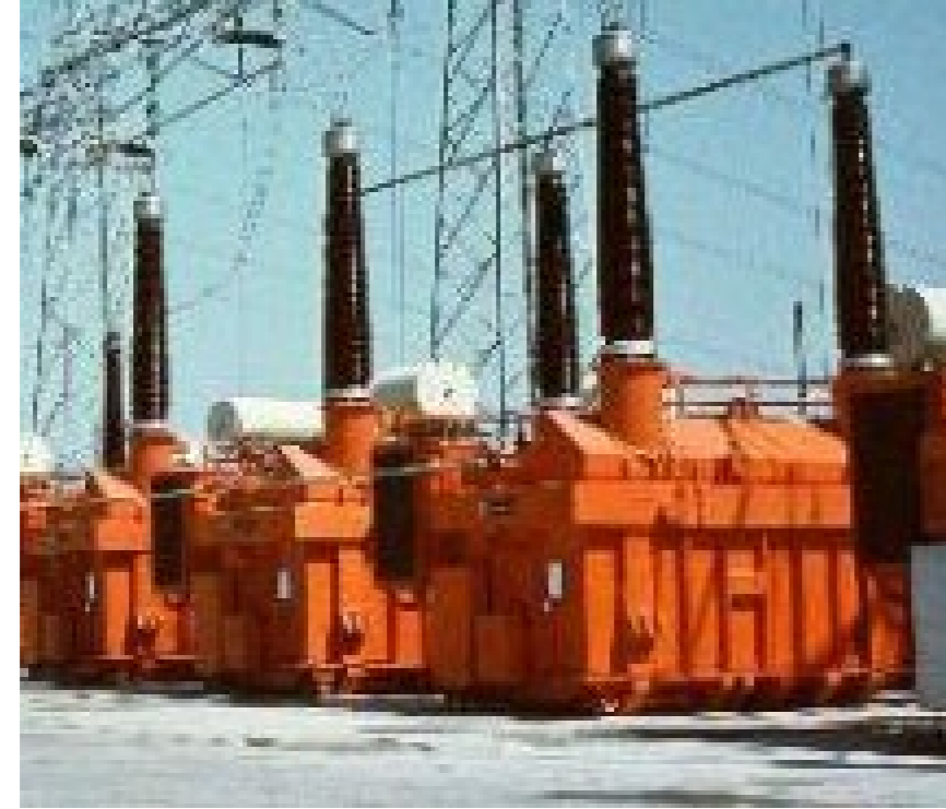
Main Power Transformers
