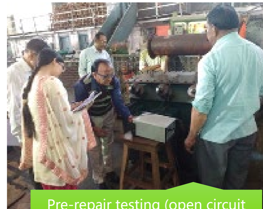
Pre-repair testing (open circuit and short circuit test) at MTRU with MPPKVCL representatives
