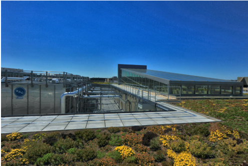
The Thomas P. O'Neill, Jr. Federal Building in Southwest DC earned LEED Platinum certification in 2014.
