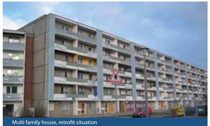
Multi family house, retrofit situation
