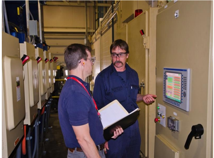
Efficiency Vermont's Account Manager reviews the performance of Husky's pumping system optimization project. Image courtesy of Husky Injection Molding Systems.
