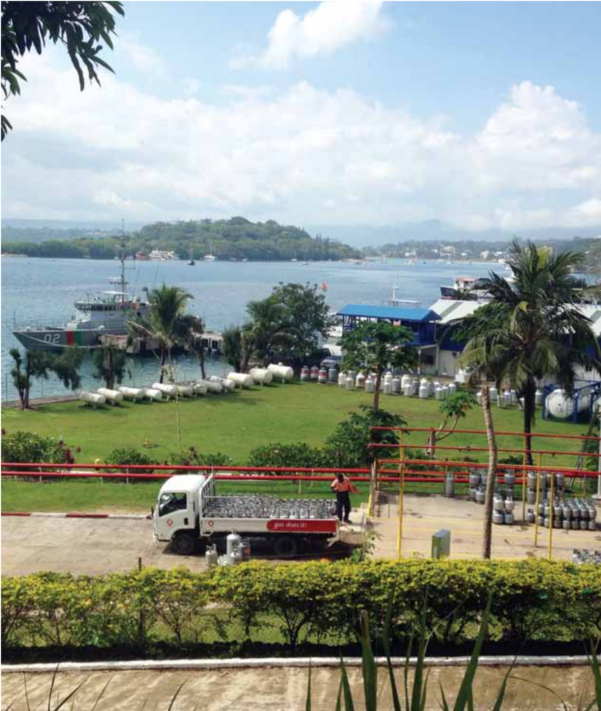
Origin LPG depot, Port Vila Photo: H. Wade
