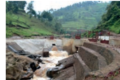
Rwanda, Photograph: REPRO Ltd.
