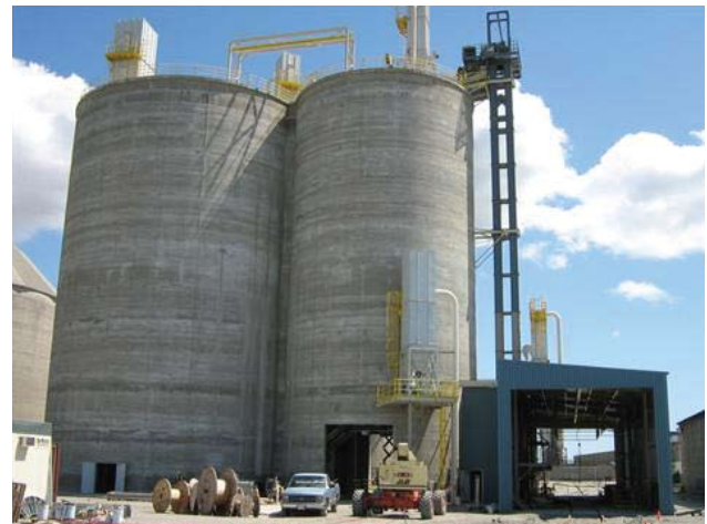
Figure 2: Fly ash silo at an Indian Cement Plant
