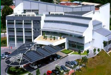
Building Integrated Photovoltaic Technology Application – Malaysia Green Tech Corporation
