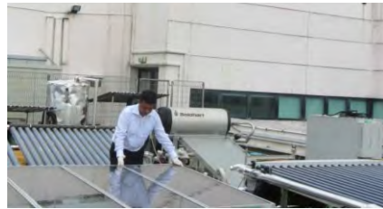
Solar collectors testing lab
