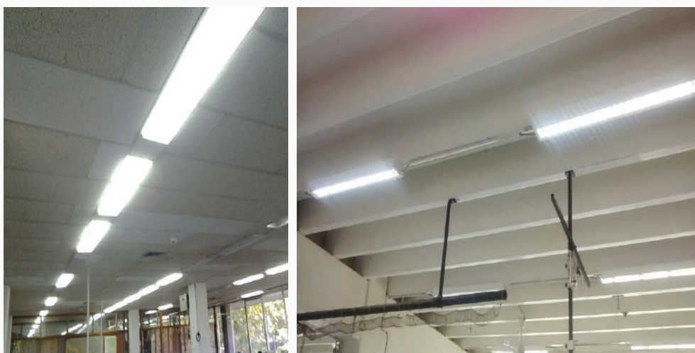
Figure 5.66: New Lighting Installation at PPL Head Office
