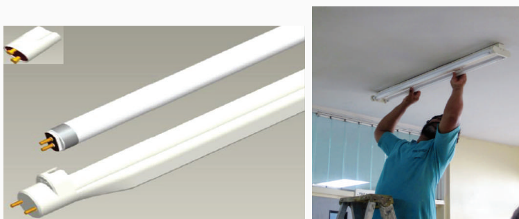
Figure 5.72: Installation of T5 Lamps
