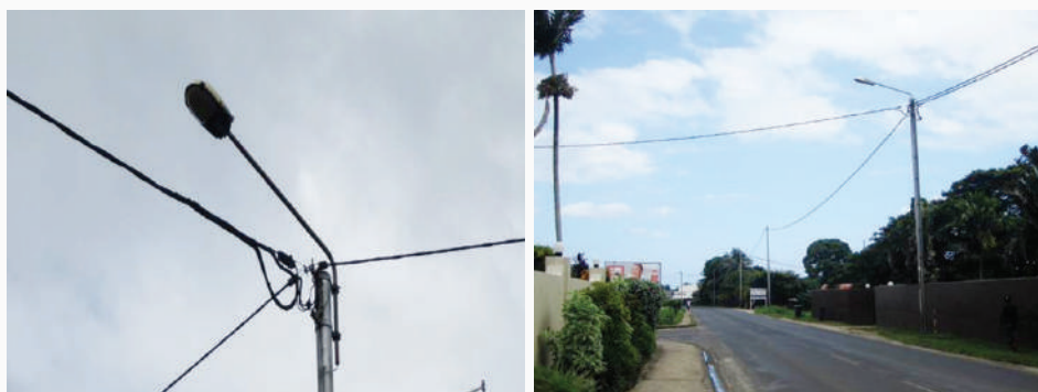
Figure 5.82: Typical Installation of Street Lighting Luminaires and Span in Port Vila
