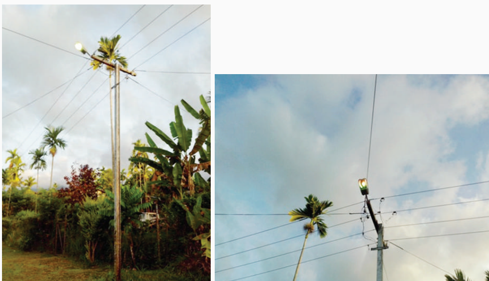
Figure 5.96: Installation of Street Lighting Luminaire in Alotau, PNG
