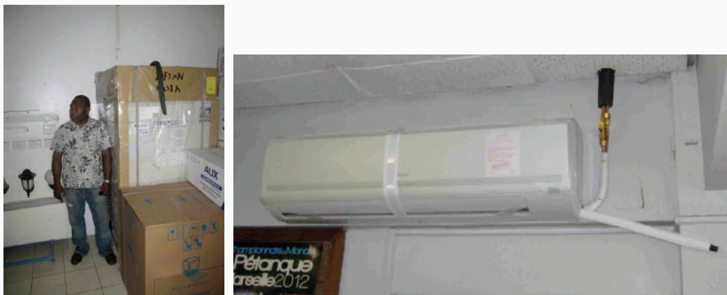
Figure 5.58: New VRF Installation at Minister's Office
