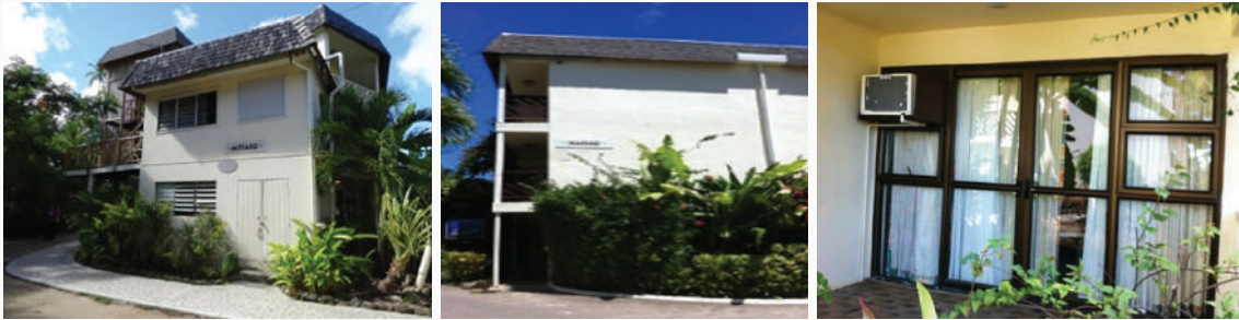
Figure 5.77: Blocks 900 and 1000 with Existing Window AC Units
