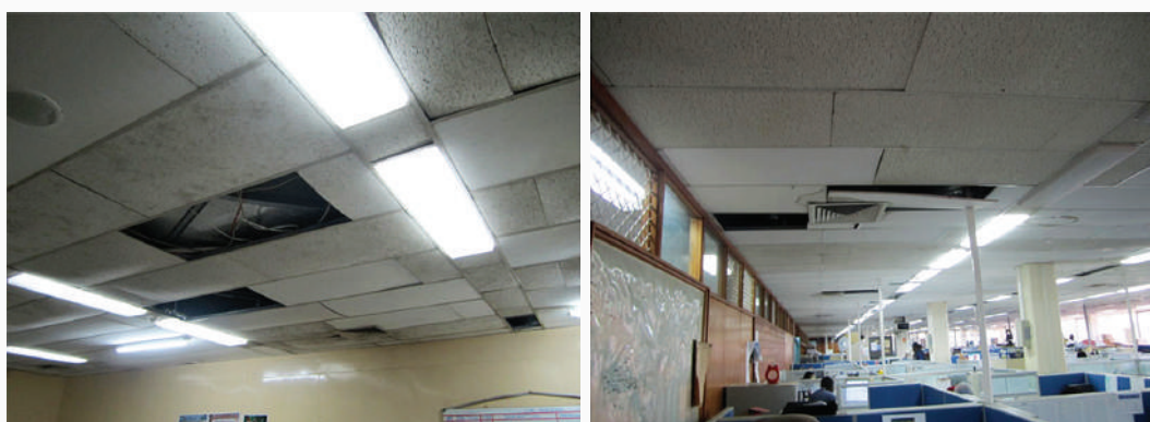
Figure 5.65: Layout of Existing Fluorescent Lamp Luminaires in the PPL Head Office
