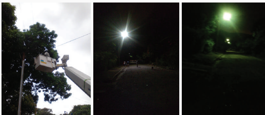
Figure 5.60: LED Street Lighting Installations in Port Moresby
