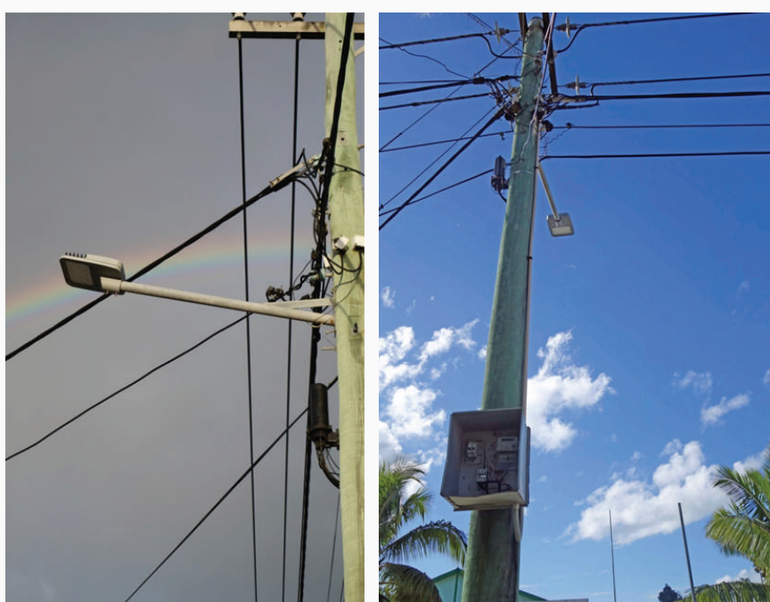
Figure 5.75: LED Street Lighting Installations in Tongatapu
