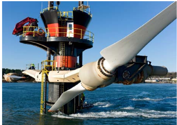
▲ Tidal stream converter under development (Strangford Narrows, Northern Ireland).
