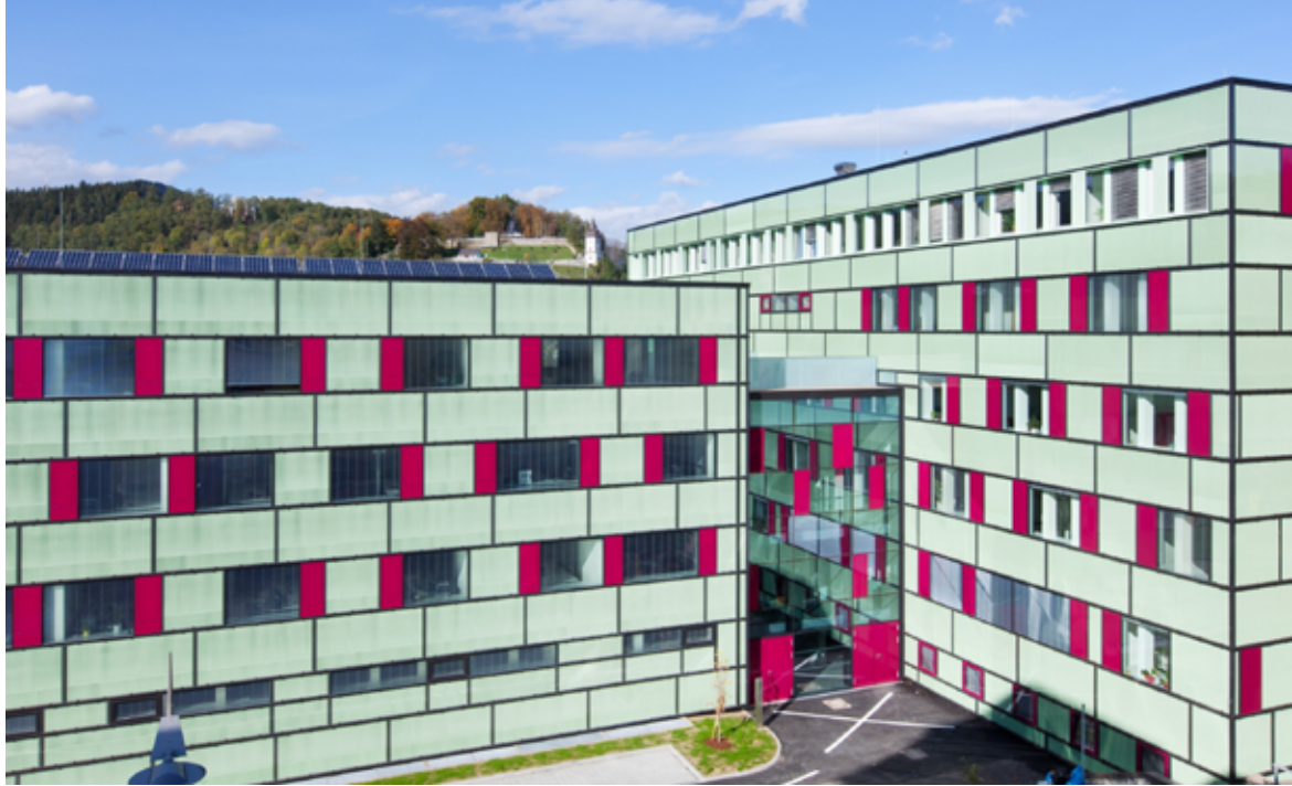
A public building in Bruck an der Mur, Austria, which includes the district court, the financial authority and the Federal Office for Metrology and Surveying - View of renovated building Source: Markus Kaiser, Graz
