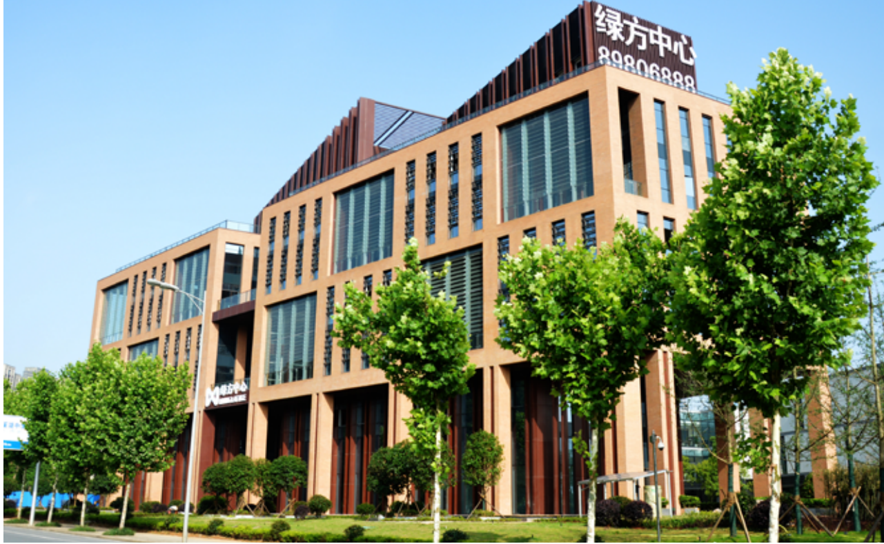
Fangxing Green Building Exhibition Center, Meixi Lake, Changsha, P.R. China. The building uses ventilative cooling though automatic window opening in mid season conditions. Source: Liang Tang
