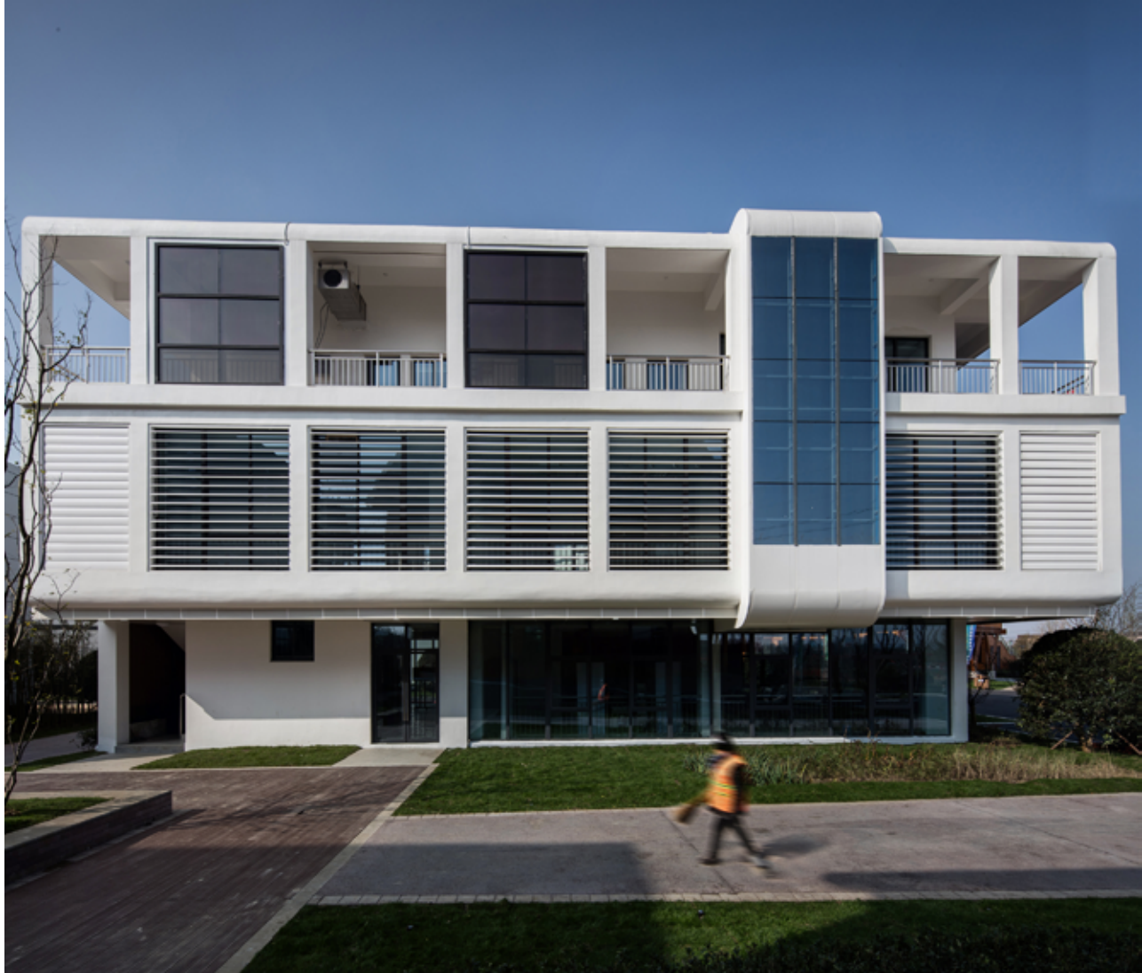
The demonstration building as a laboratory for High IAQ Low Energy Design, P+, in Changzhou, P.R. China. The building was designed by project participants and integrates a number of strategies, methods and technologies being studied during the project. Source: P+ Design Group, Nanjing University and Syracuse University Center for Green Building and Urban Environment
