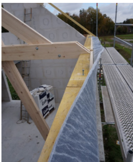
Aerogel mats installed in a single house to avoid thermal bridges. Source: Agence ARC Urbanisme and Architecture and ISOLProducts SAS
