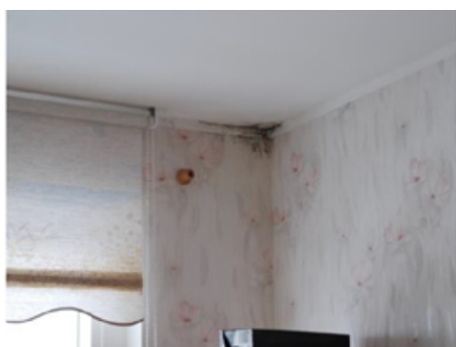
Visible mould growth at the corners of a building envelope, possibly caused by a thermal bridge.
