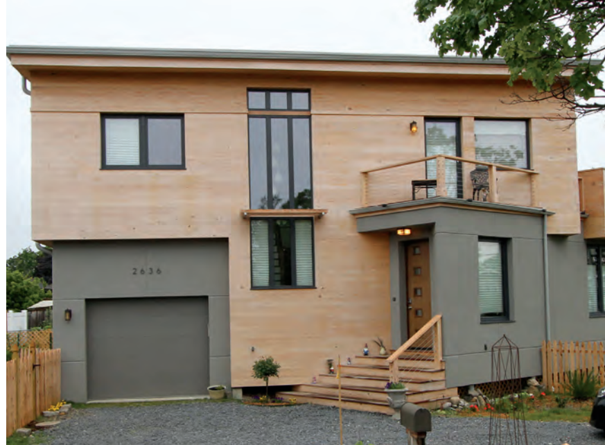
Great South Bay Passive House; Photo by Anthony Musso
