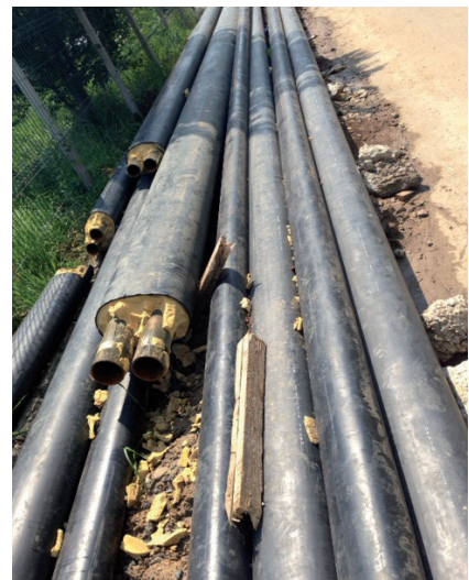
New city development in China (top). Pre-insulated district heat pipe in Botosani, Romania (bottom).
