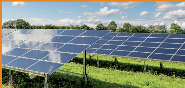
Solar photovoltaic panels in a field in Bavaria, Germany.
