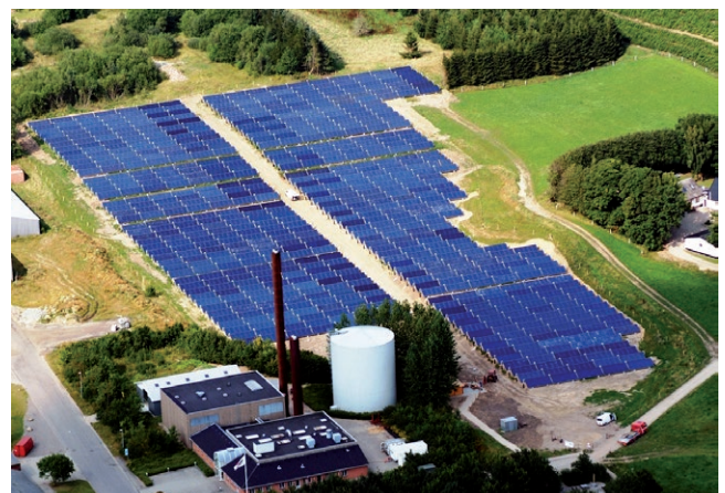
A large solar thermal plant with heat storage connects to a district heating network in Brødstrup, Denmark.
