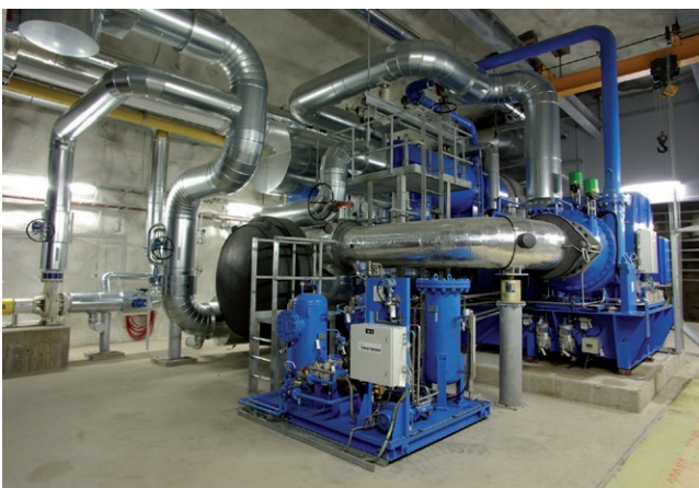
Helsinki’s Katri Vala heat pump captures heat from the city’s waste water.
