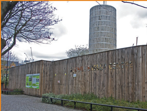
Bunhill CHP plant in Islington, London. The tower is a large heat storage unit that reduces the need to provide heat from the district heating system's backup gas boilers.
