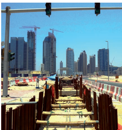
Laying district cooling pipes in Dubai, UAE.
