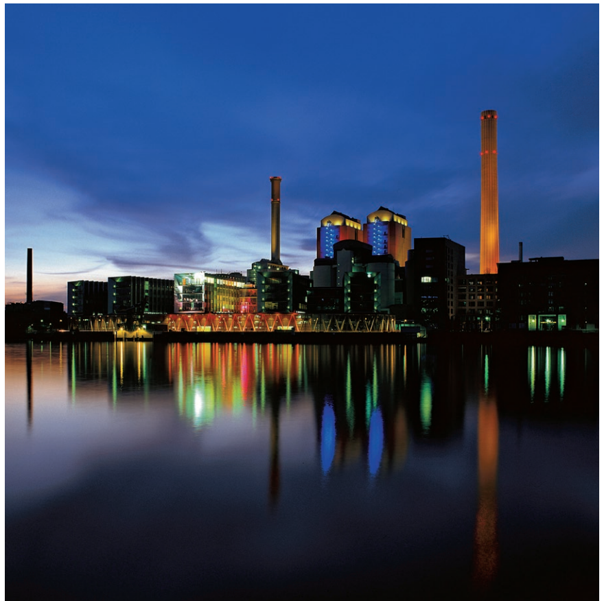
Heizkraftwerk West CHP plant in Frankfurt, Germany.
