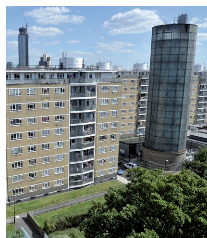
A glass accumulator tower at Pimlico District Heating Undertaking in London stores excess heat from the network.
