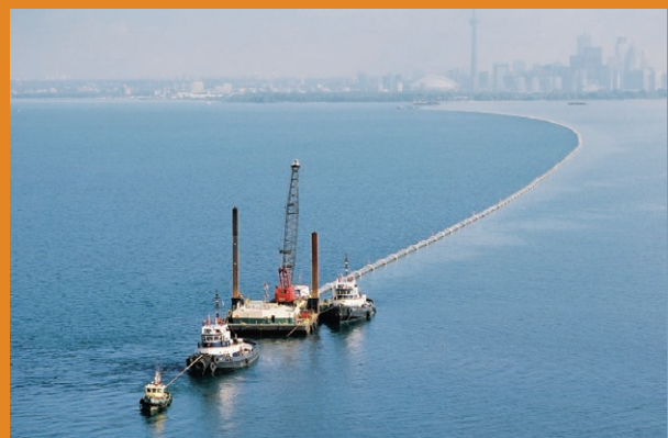
Toronto's deep-water cooling system captures cooling from Lake Ontario (see case study 3.5).
