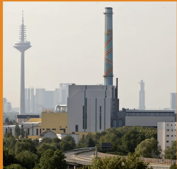
Waste incineration plant in Frankfurt's Nordweststadt with a capacity of 525,000 tons per year.
