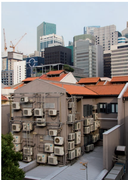
Air-conditioning units on a house in Singapore, 2013.
