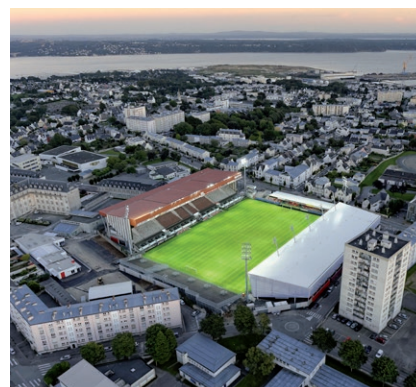
Oslo, Norway (top). Stade Francis le Blé in Brest (bottom). Connecting stadiums, leisure centres, hospitals and other anchor loads diversifies the load, making the district energy system more efficient.
