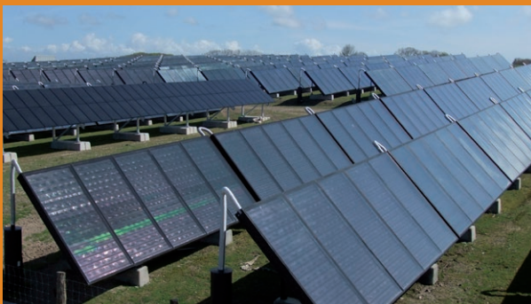
Solar thermal plant (left) and CHP plant (right) in Sonderborg.
