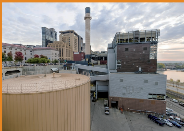
Wood chip CHP plant in St. Paul, USA.
