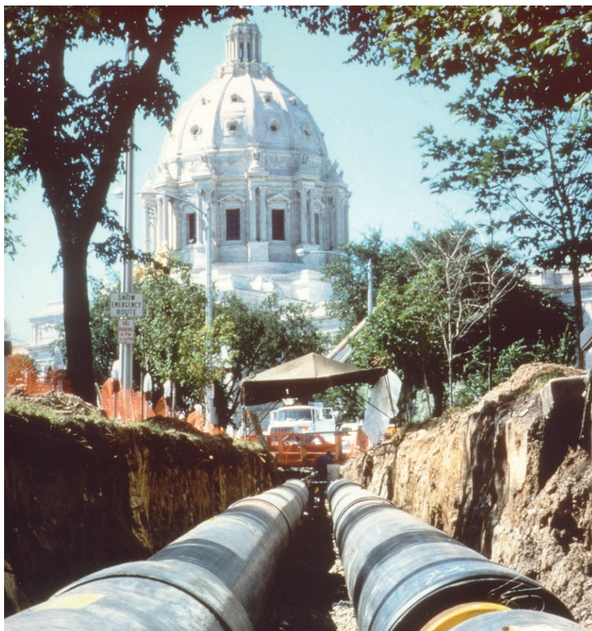
Laying a section of St. Paul's district heating network in 1982. The network heats 80 per cent of downtown buildings, including the Minnesota State Capitol, seen in the background.
